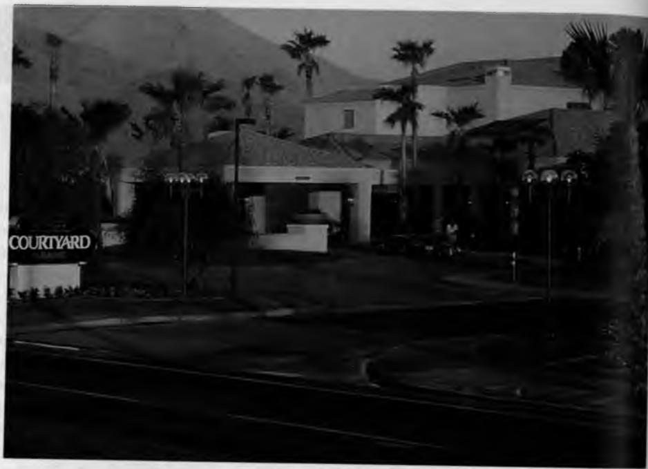
Courtyard by Marriott. Courtesy of Marriott International, Jim Burnett, photographer.
