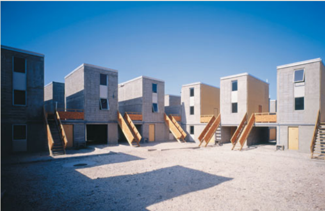
Alejandro Aravena's 2001 low-cost housing project, Quinta Monroy in Iquique, Chile, introduces an aggregation of standard concrete units that are intentionally incomplete,
