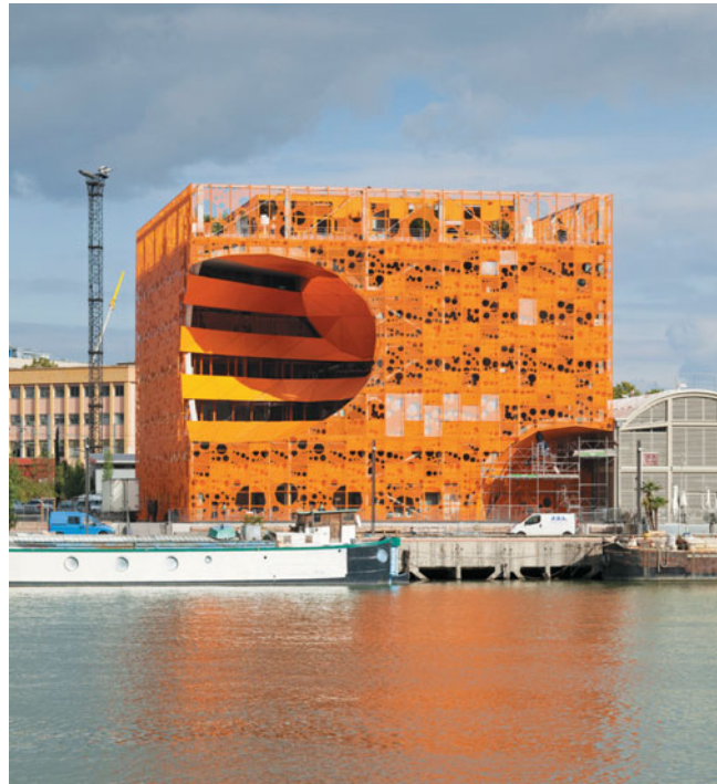
The Orange Cube in Lyon, France by Jakob + MacFarlane Architects (completed 2011), achieves the effect of considerable depth of surface by layering a perforated
